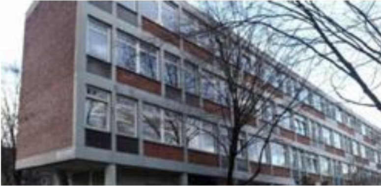
RC frame, masonry in-fill and shear walls
