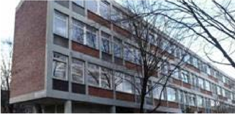
RC frame, masonry in-fill and shear walls
