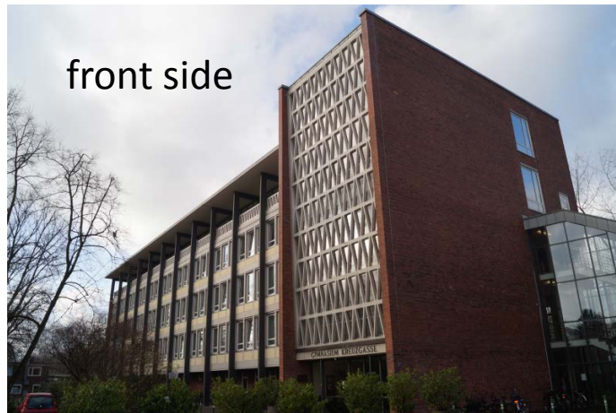
RC frame, in-fill walls, shear walls
